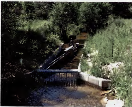
Figure 36. Self-cleaning fish screen.
